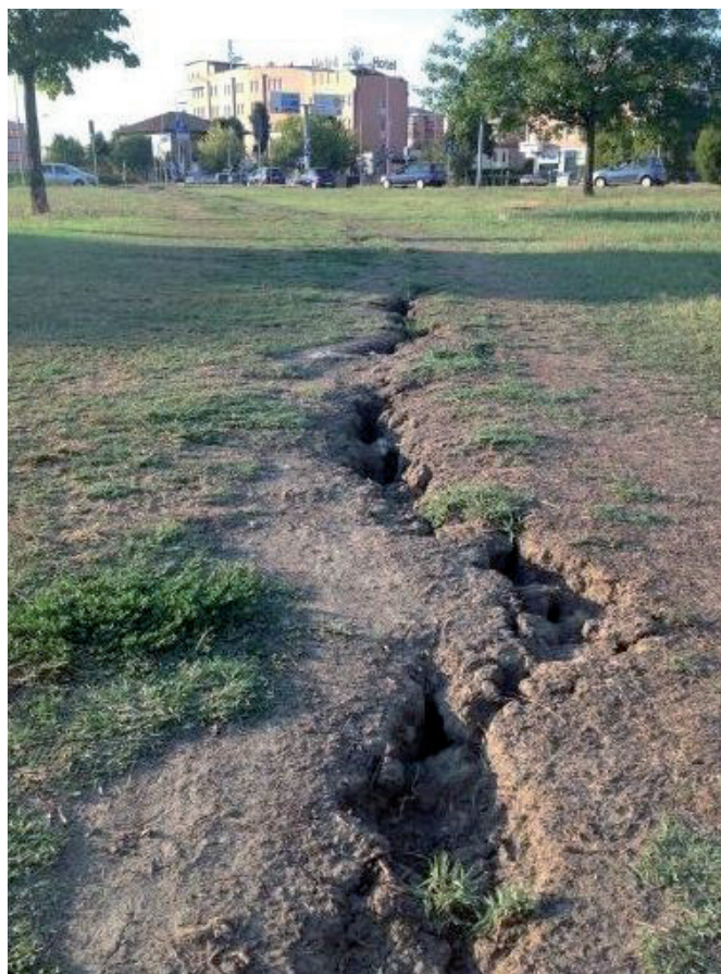
Fig. 10 - 20 m ground fracture which appeared in Ferrara in August 2013 (courtesy of Dorianò Castaldini).
